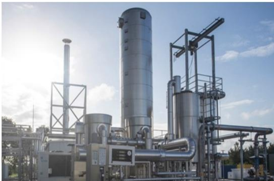
Fig. 2 Power-to-Gas Plant to Produce E-Gas (Source: Audi AG)
