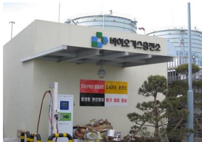
Fig. 3 Biomethane Charging Station
