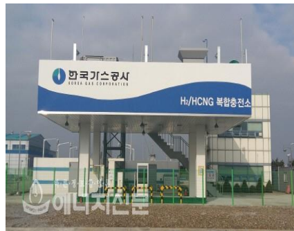
Fig. 2 KOGAS H 2 /HCNG Station
